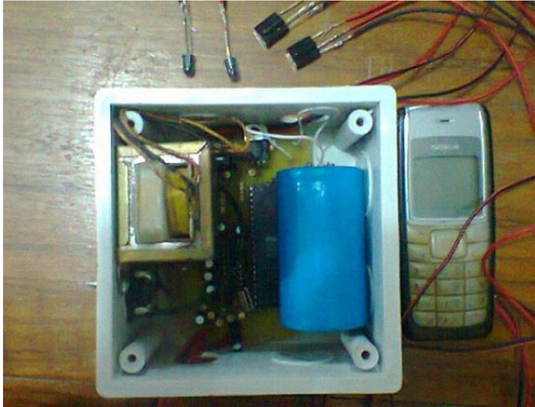
Plate 3.1: Casting of the SMS based burglar monitoring system
