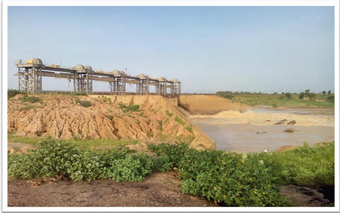
Plate I: Gated Channels of Yardantsi Reservoir as Outlets for Flood Control
