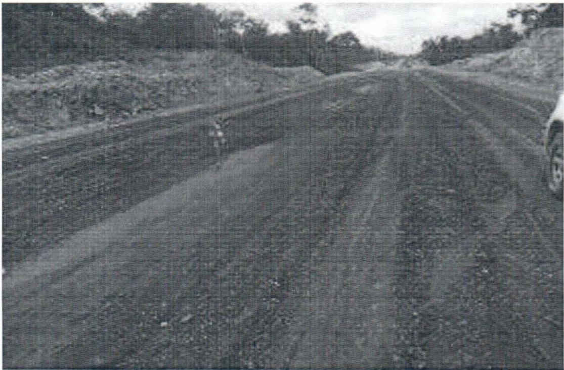
Pictorial Illustration 2 Construction of Road in a community in Akamkpa
