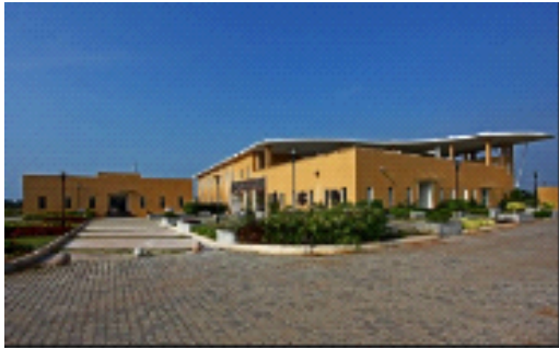
Figure 11 Main Building Entrance
