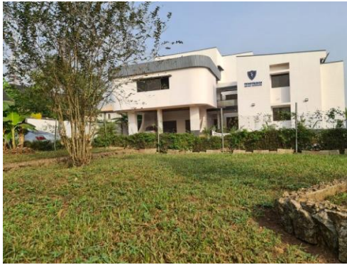
Figure 13: Front view of building
