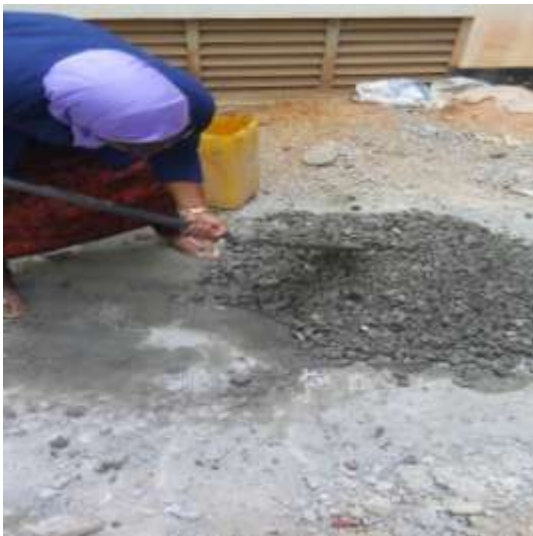
Plate VII: Hand mixing of Aggregates
