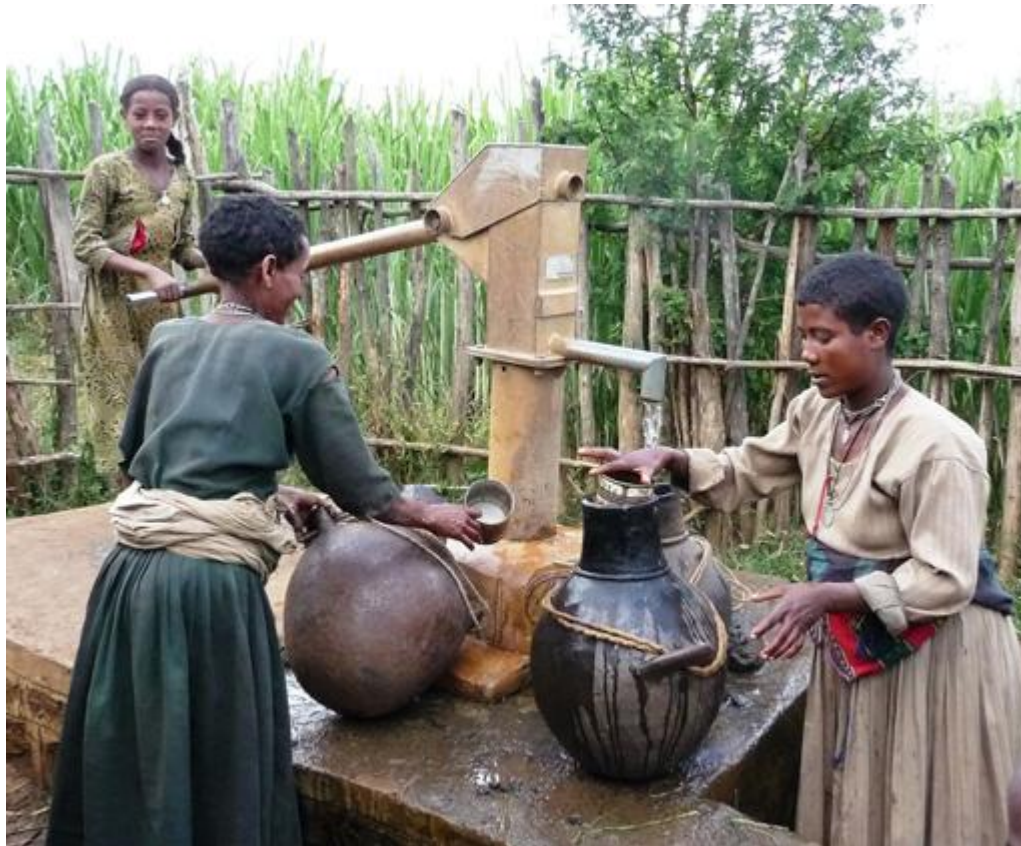
Plate: 3 Borehole with manual hand pump
