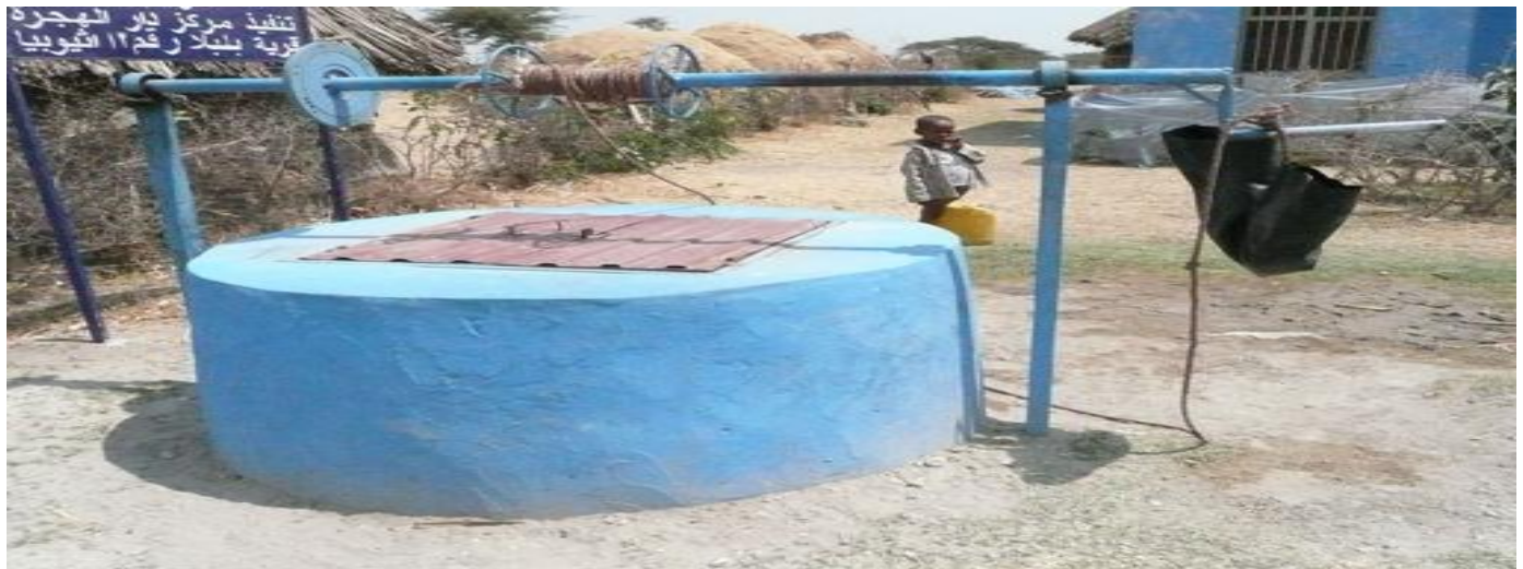
Plate 1: Hand pump over a protected dug well
