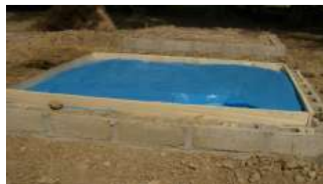
Plate 3.5: Foundation insulation
