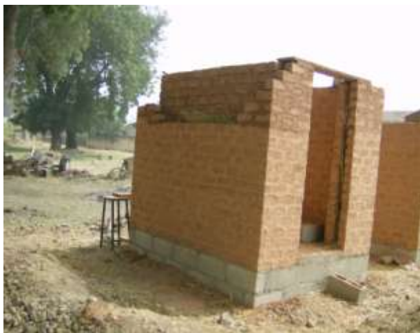
Plate 3.7 : Room under construction
