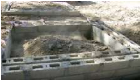
Plate 3.4: Hard core foundations installation
