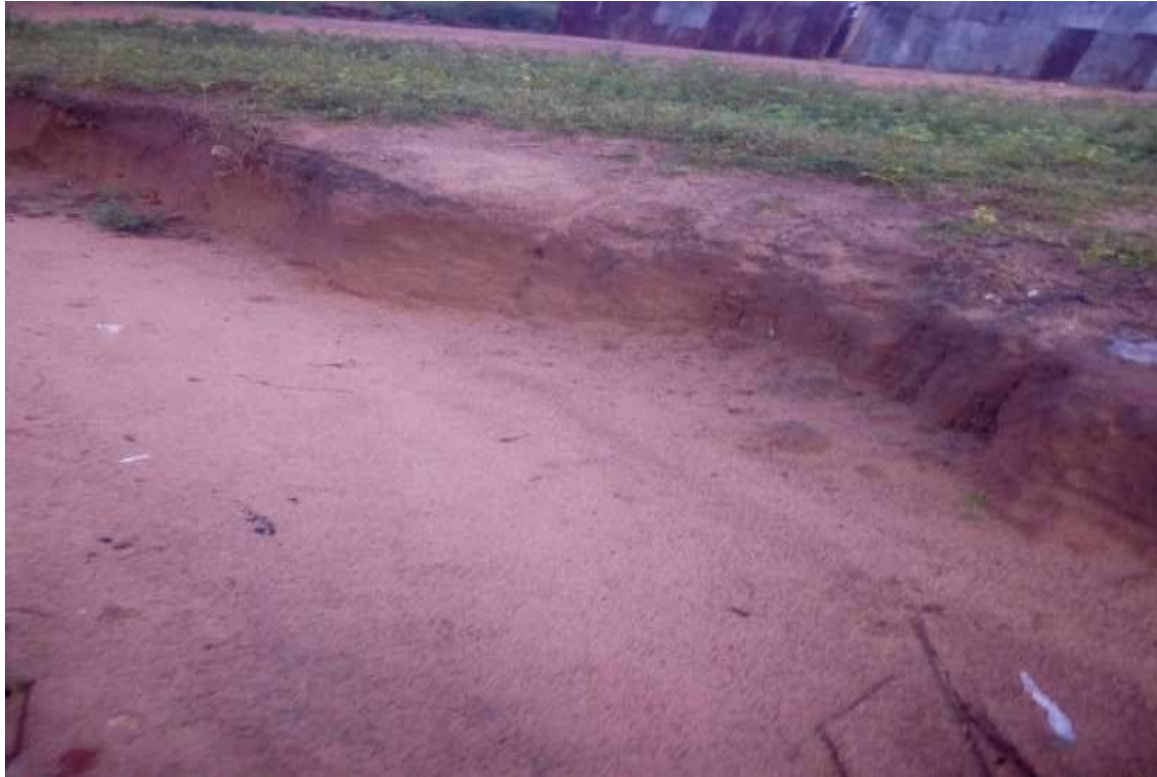
Plate 1: Eroded Farm in kpotegi Community (Gulu distict)
