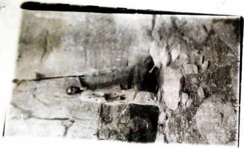
PLATE 1. SHOWING JOINTS IN GNEISS
