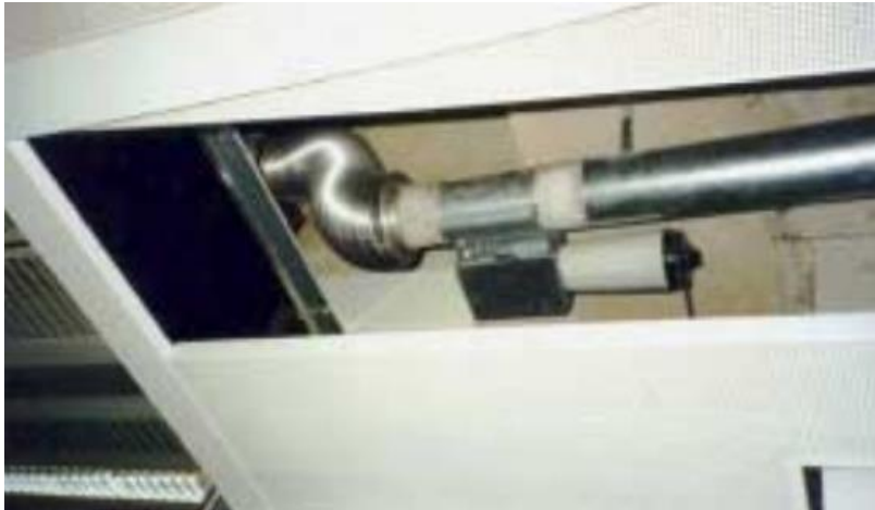
Plate XII: Distribution Ducts and Control Facilities in an Easy-to-Dismantle Ceiling. Source: CIB World Building Congress, 2015.
