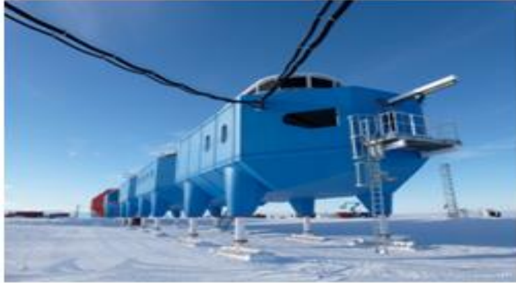
Plate VI: Mobile Home for 50 Scientists, Hhalley Antarctic Research Station. Source: Hugh Broughton Architects, 2015.
