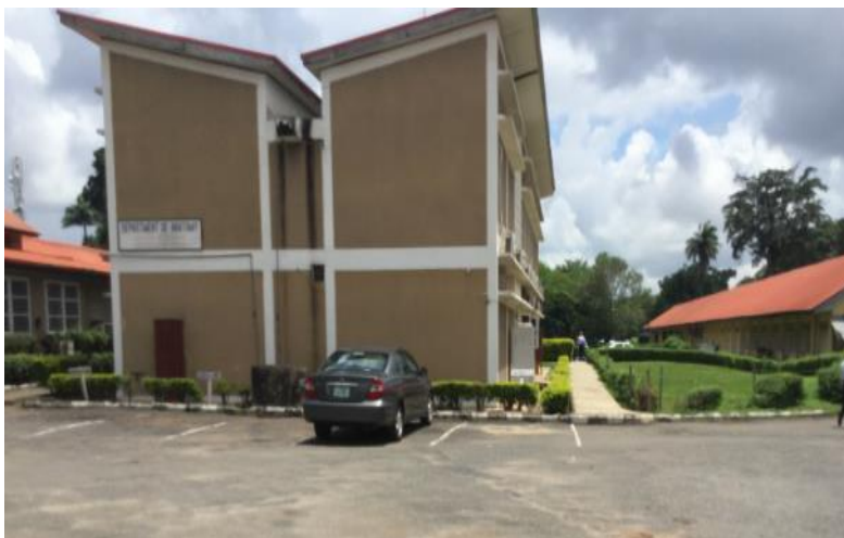
Plate XLI: A View of the Faculty of Medicine U.I, Showing the Building Form Adapted. Source: Author's fieldwork, 2016
