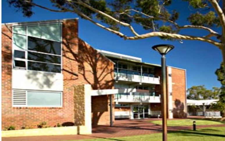
Plate XIV: Scotch College Upper Primary Boarding House Recycled. Source: OECD, 2016.
