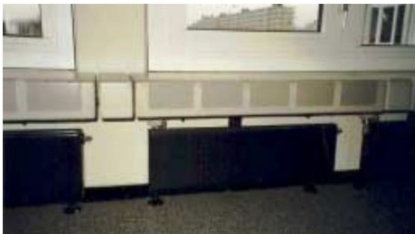
Plate X: Modular Radiator and Window ledge System with Dismountable Walls. Source: CIB World Building Congress, 2016
