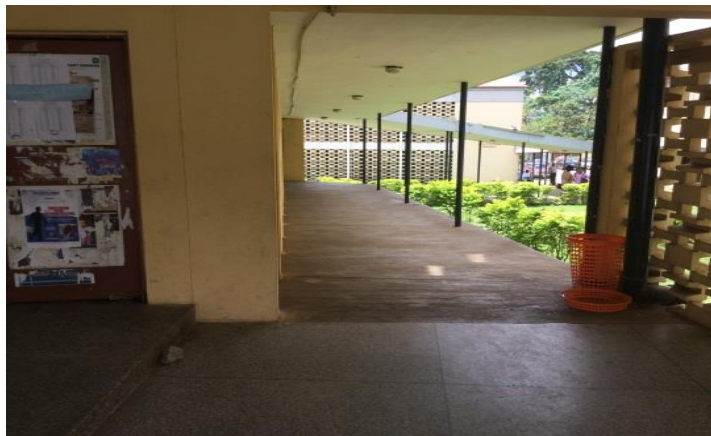
Plate XLII: The Faculty of Medicine U.I, Having Interconnection between Spaces. Source: Author's fieldwork, 2016
