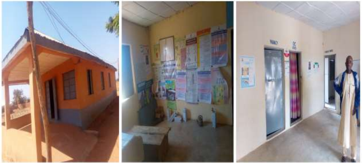
Health post center constructed by the CSDP in Maigwaza and Gidan Illo Community of Kebbi and Zamfara States respectively
