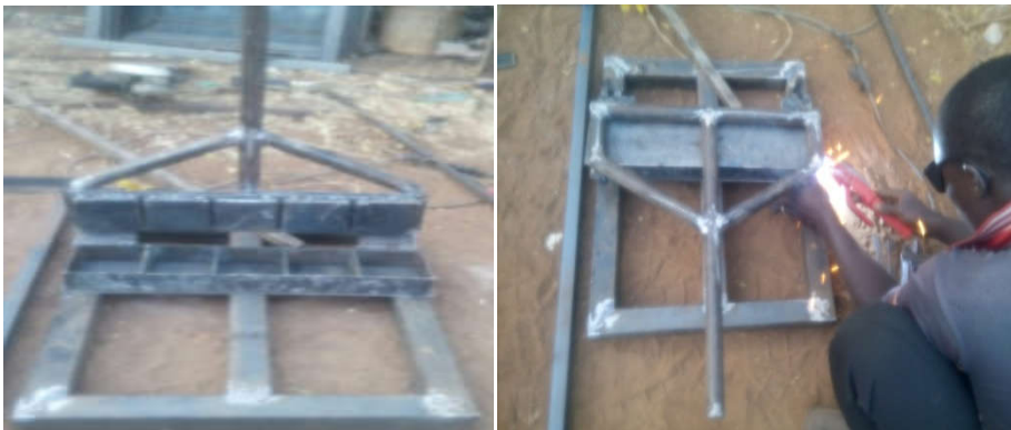
Plate IV: Briquette moulding machine under construction
