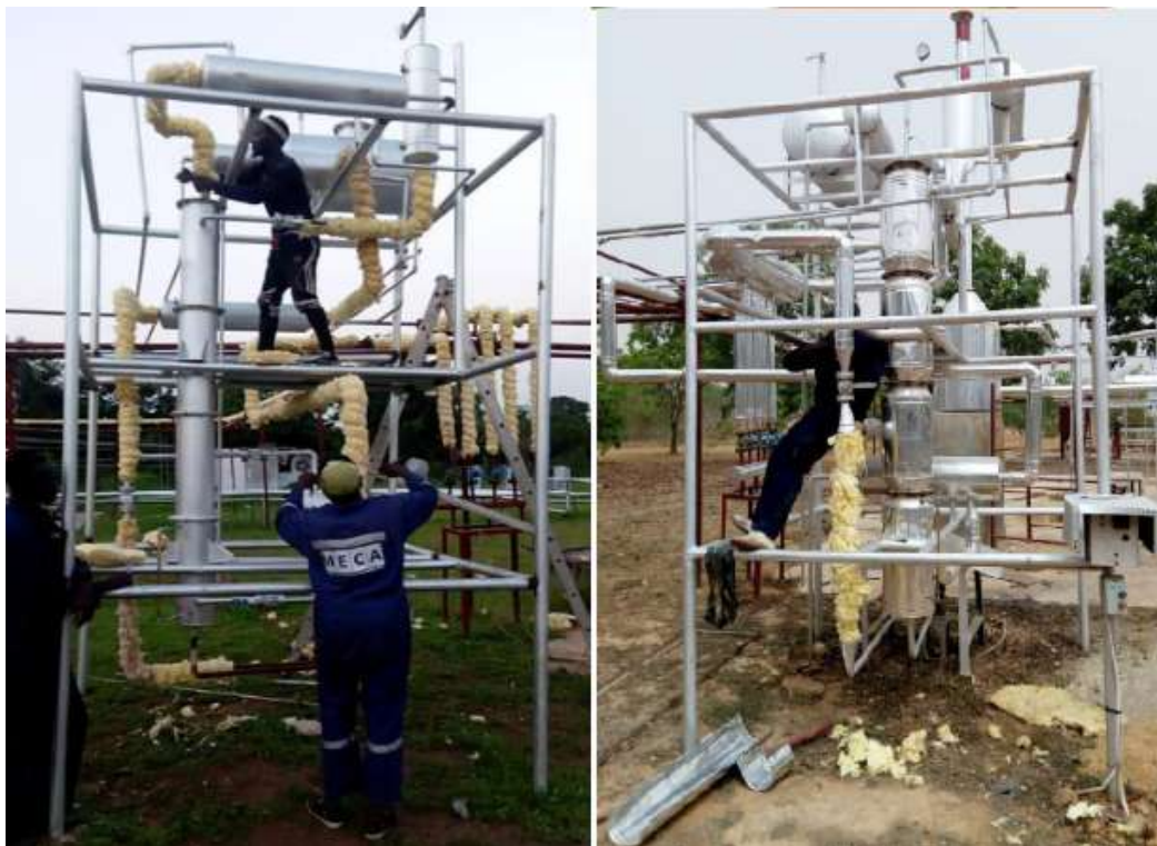
Plate 4.8: The installed SWS Unit during Lagging
