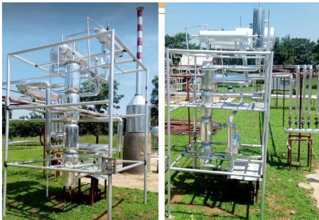
Plate 4.8: The installed SWS Unit during Lagging
