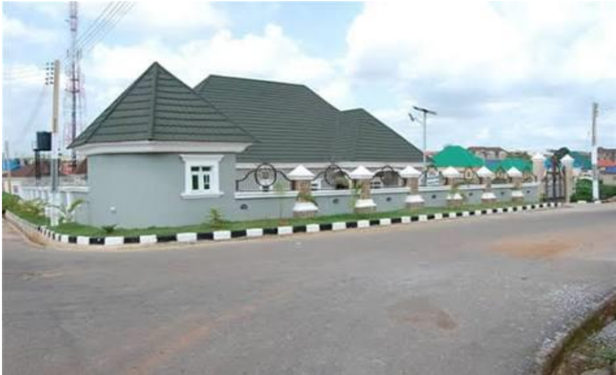
Plate 1 showing Efab Housing Estate located at Lokogoma.
