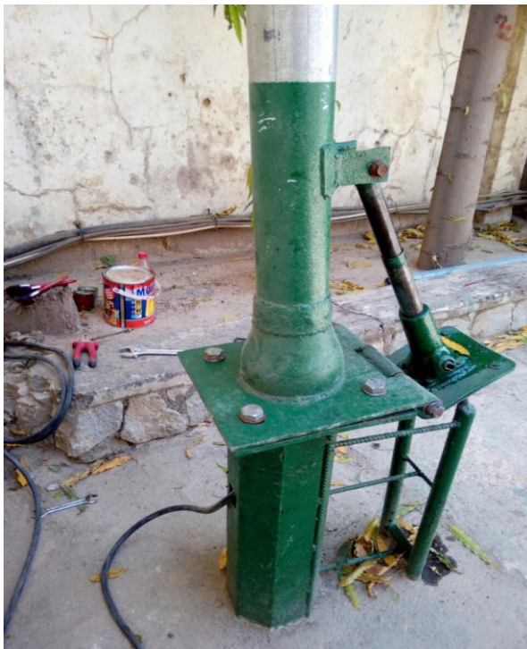
Plate A IV . Self-erecting part after commissioning
