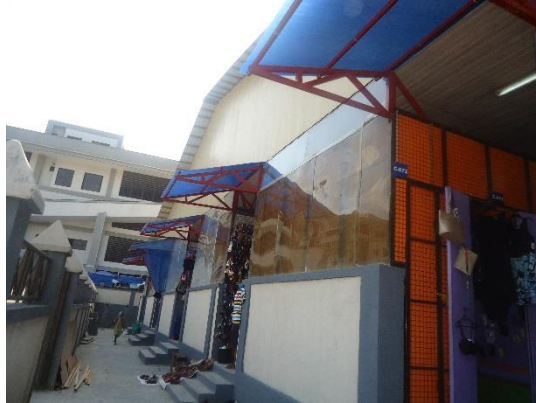
Plate XXII: View of ingress into single unit structure
