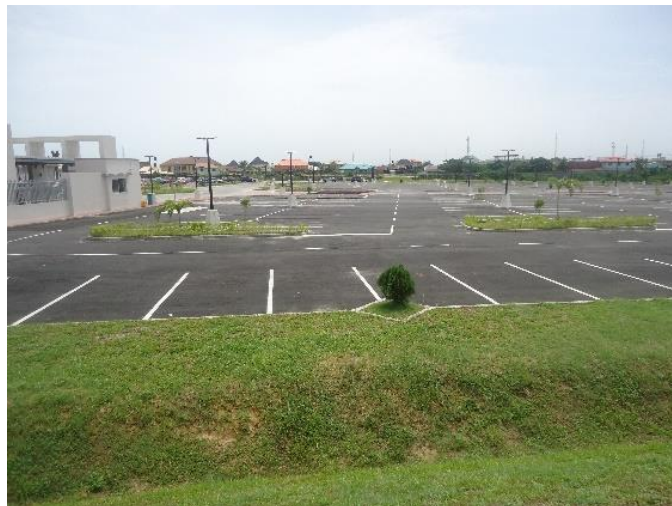
Plate I: View of large parking lot.
