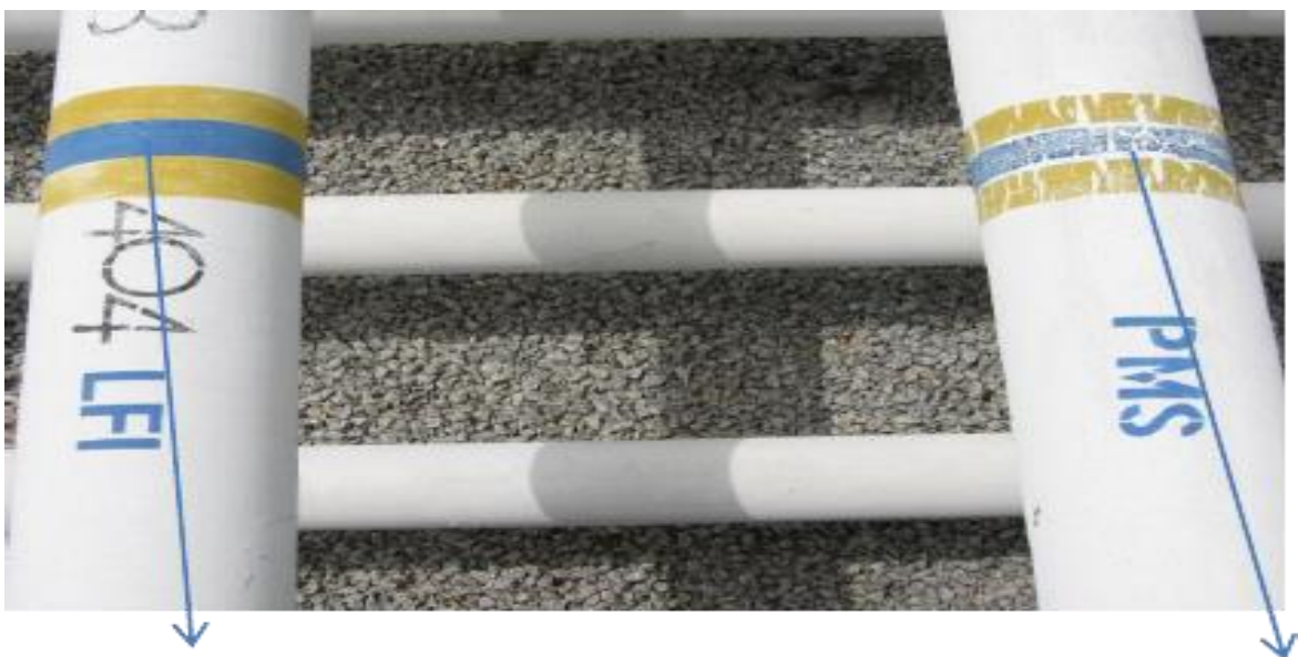
Plate 4: PPMC Pipes for various Crude oil Products at Sarkin Pawa Pump Station
