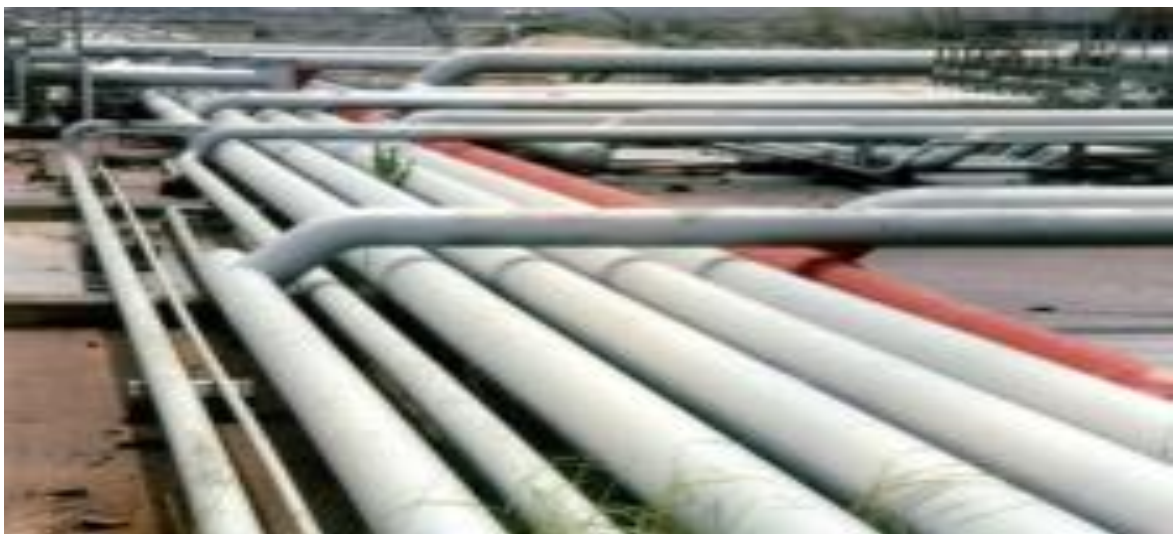
Plate 6: PPMC – NNPC Pipes for transferring of various Crude oil Products
